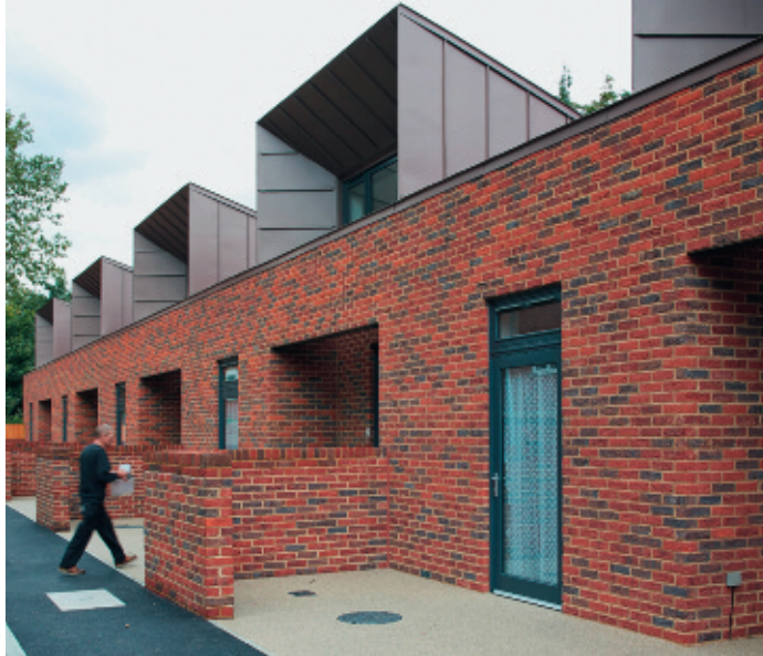
Foto nº 23. Greenwich Housing https://www.dezeen.com/2015/11/16/bell-phillips-architects-brick-mews-zinc-clad-roofs-cost-effective-housing-greenwich-london/
