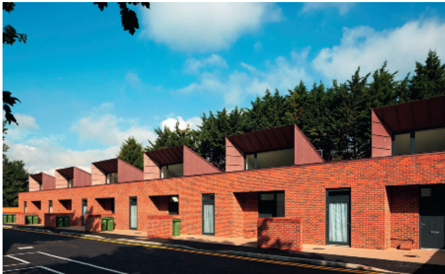
Foto nº 24. Greenwich Housing https://www.dezeen.com/2015/11/16/bell-phillips-architects-brick-mews-zinc-clad-roofs-cost-effective-housing-greenwich-london/
