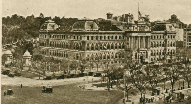
MINISTRY OF PUBLIC WORKS (Madrid)
